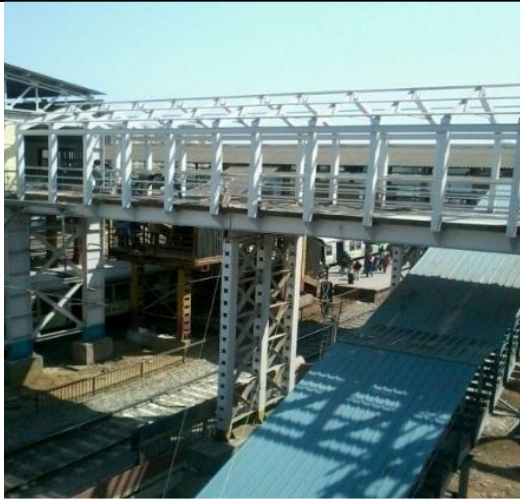
Construction of foot Over Bridge
