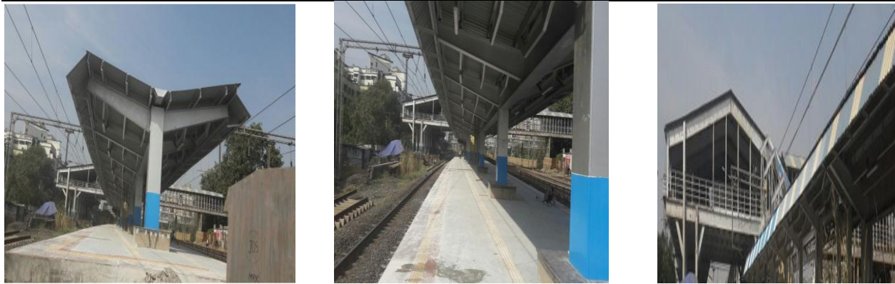
Construction of FOB's, Booking Office & Platform
