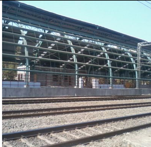
Construction of PEB Platform
